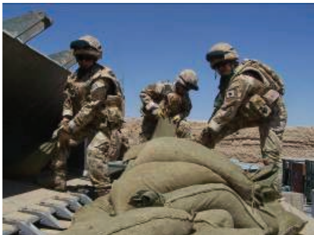
Reinforcing a roof with sandbags
