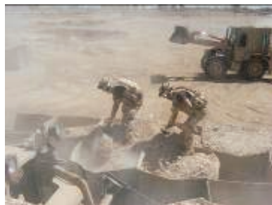
Filling HESCO cells on a FOB wall
