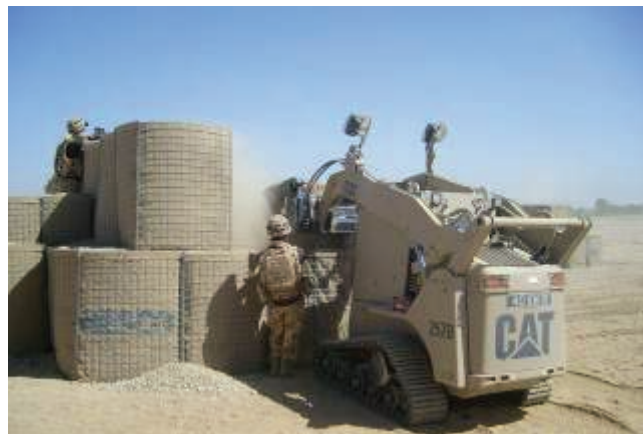
Mini digger assisting with sanger construction
